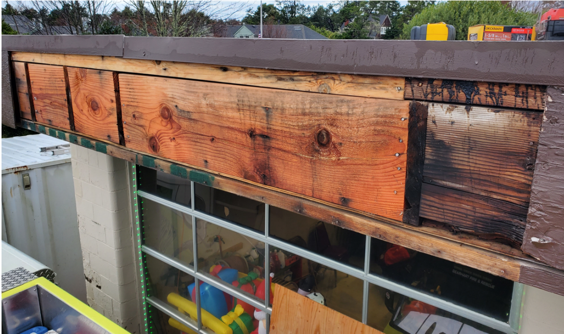
Figure 6: Exterior view of Framing
