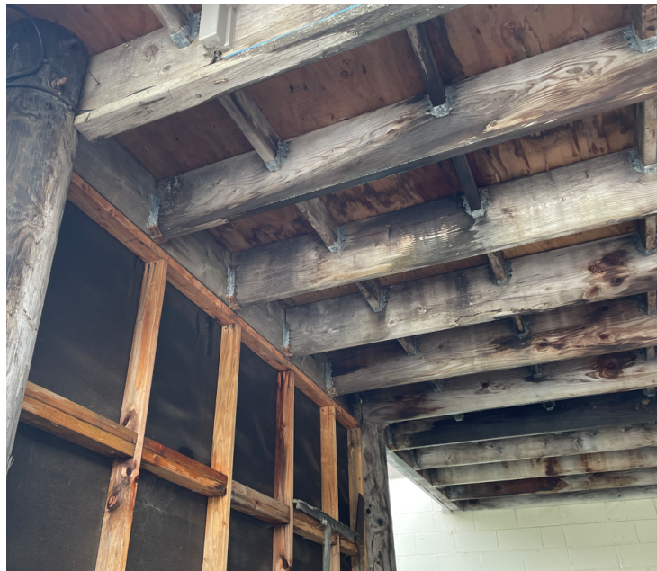
Figure 7: Exterior Canopy Framing
