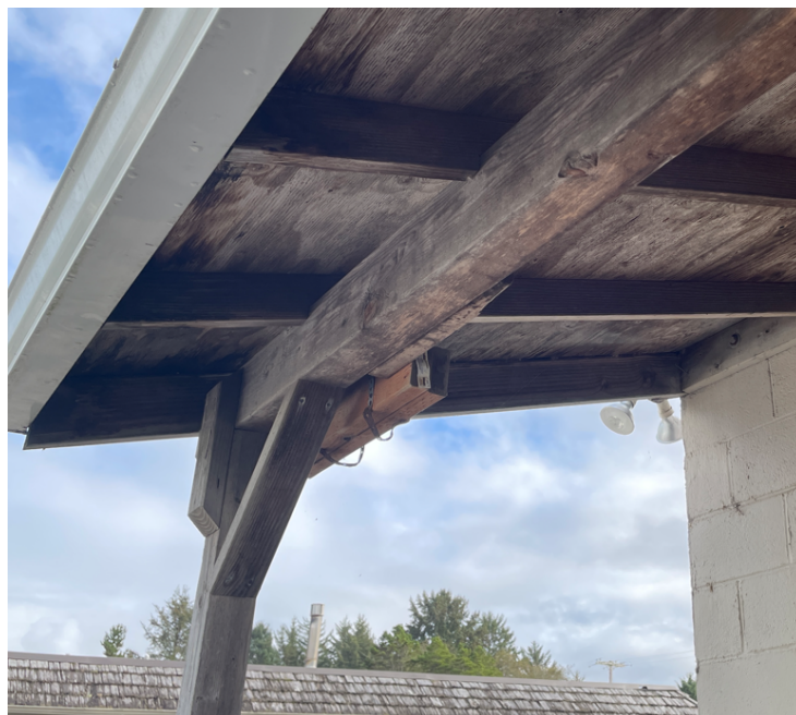
Figure 8: Exterior Canopy Framing
