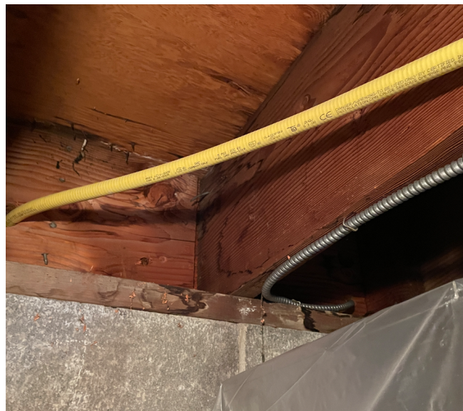
Figure 5: Roof Framing Sill Plate
